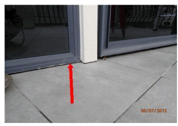
64) VISIBLE FLOOR BASE LEAKING
